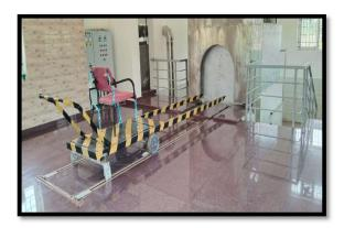
Under the mission, Electrical crematorium is constructed which is for all class of the people. The project components include AWL Cremator, Combustion Air supply system, Wet Scrubber (Vane type), Stack (Self supported), Control Panel, Manual "Dead Body" charging systems and the **Dead body cremation will be** 1 body/hour.
